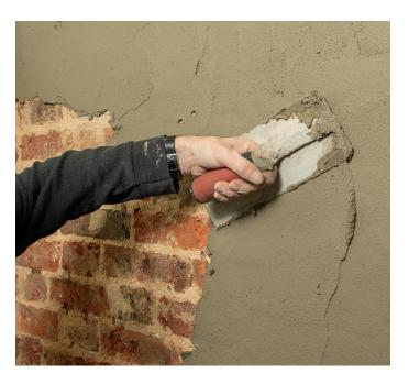
Dryzone® Fast-Set Plaster is designed to set within 2 hours at 20 °C. In colder temperatures the set will be slower but can be accelerated by using warm water. In hot temperatures the set will be faster and can be slowed using cold water.
