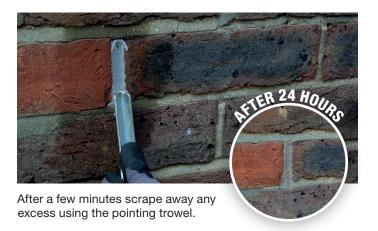
**Stormdry® XR-Mortar** cures by evaporation of moisture. In cold and damp conditions this drying process can be slowed, especially when applied in thick layers. For thick applications it may be necessary to apply the mortar in two layers to achieve an even cure. When applying the second coat push the mortar into the first coat for a good bond.
